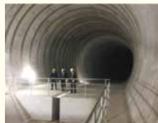
Shirako River Flood Control Reservoir (Capacity: 212,000 m 3 ) Structure type: Underground tunnel Accumulation rate during Typhoon Hagibis: Nearly 90%
