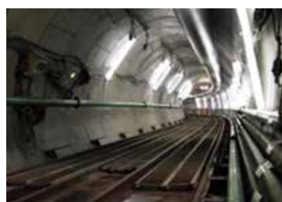
Second Tagara River Mainline (under construction)
