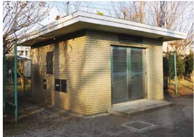
Management facilities of emergency water tanks within Gakuden Park. (A 1,500-sq. m water tank is located below ground.)
